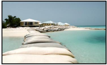
Photo 15. A view of GeoBags forming beach groins and revetment at the Anegada Seaside Villas.
