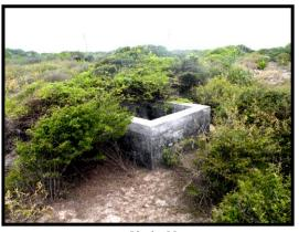
Photo 11. Typical freshwater well on the Limestone Plain. Concrete sides are to protect the sinkhole from filling up with rock debris and animal residues.
