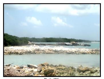
Photo 124. A series of landfill groin structures east of Setting Point. Access necessitated clearing through the fringing Red Mangrove forest in the background.
