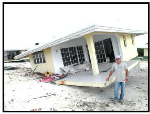
Photo 8. Many cottages along West End Point are at risk and have become vulnerable due to severe beach erosion.
