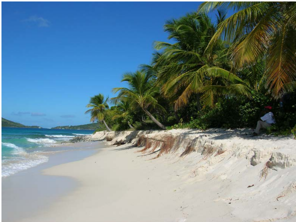
Photo #4: Erosion along western shoreline has downed a few palms trees.
