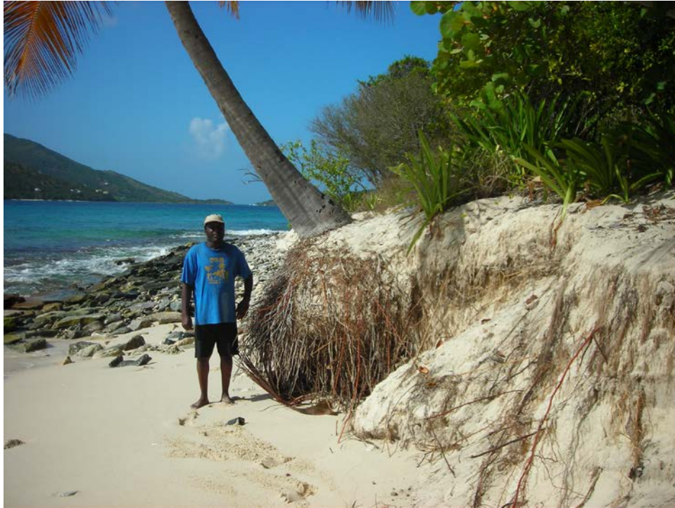
Photo #3: Mr. Blyden standing in front of an eroding shoreline bluff and tilting palm tree.
